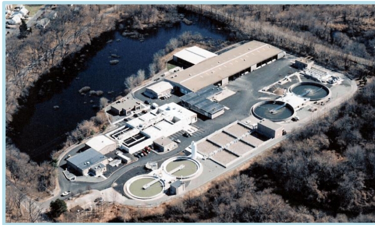
West Warwick Regional Wastewater Treatment Facility
